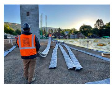
Also known as a vapor mat, these passive radon mitigation systems are primarily used in new construction. An extremely strong pressure-resistant plastic membrane is placed directly on the soil prior to the foundation being poured. This allows for radon to move freely under the concrete foundation and be passively vented outside without the need of a fan.
