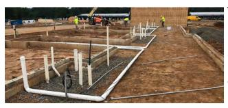
The most common form of radon mitigation in commercial structures is sub-slab depressurization (SSD). SSD systems work by generating negative pressure under the slab of a structure to draw rising gases out before they have a chance to get in.
